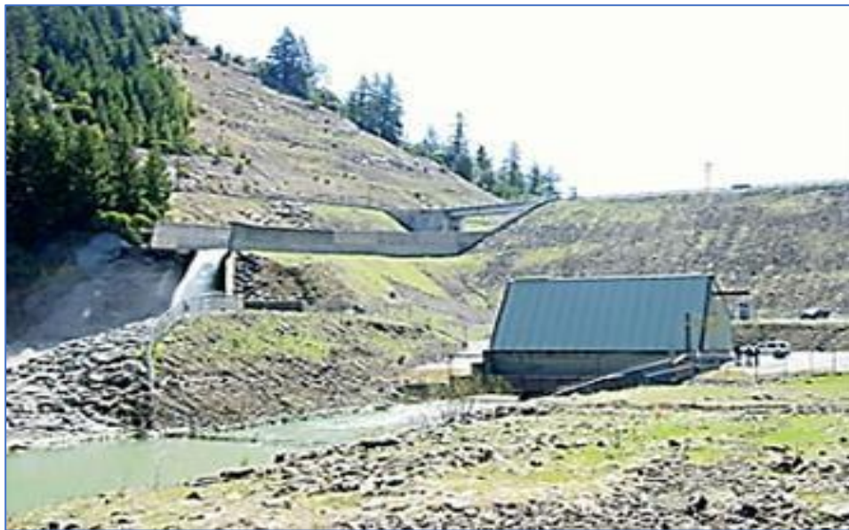
Figure 4.9: R.W. Matthews Dam near Ruth
