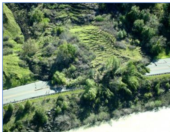
Figure 4.14 Landslide along US 101
