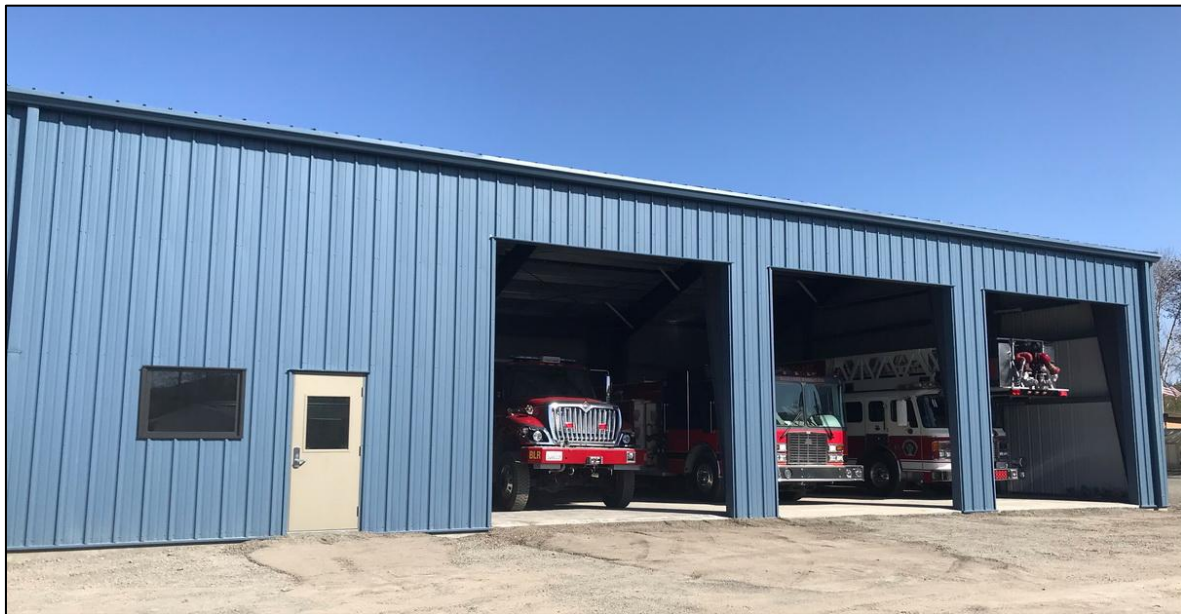
Figure 3.6 BLR fire station shown under construction in April 2021.
