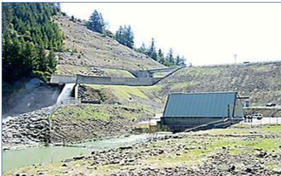
Figure 4.9: R.W. Matthews Dam near Ruth
