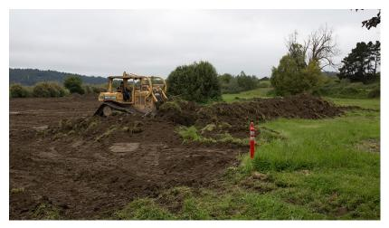
Kernen Heavy Equipment Operator Aaron Ashcorn begins grading the construction site in preparation for the installation of Blue Lake Rancheria's 500-kW solar array. Photo from Blue Lake Rancheria
