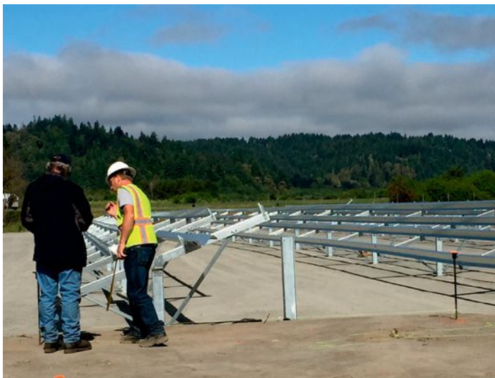
Workers installing the racking for the Blue Lake Rancheria’s solar system.
