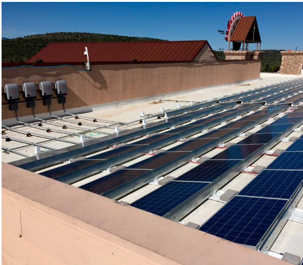
A 75-Kw solar PV array installed on the Tonto Apache Tribe's Tribal Administration Building as part of a 2014 project co-funded by DOE. The tribe anticipates saving an estimated $1.8 million in energy costs over the project's projected 30-year lifespan.
